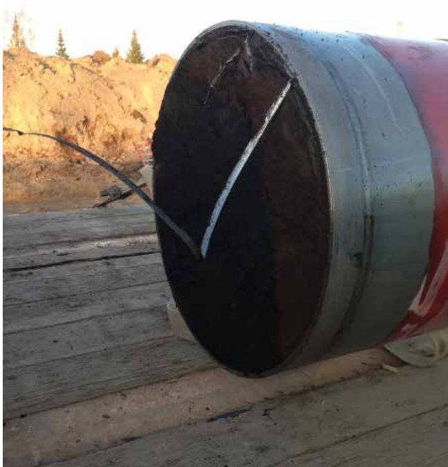
Figure 6. Cross section of pipe showing extent of blockage.
